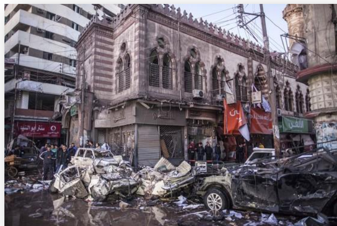
Figure 1.1: Devastation caused by a bomb attack in Mansoura, Egypt
